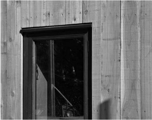
**Fig 8. Rainscreen of rough sawn cedar planks on the Totnes house.**
