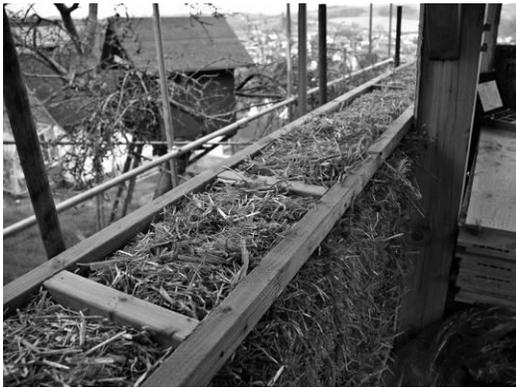
**Fig 6. 'Ladder' made from 38x38mm batten, laid on the second course of bales, provides a valuable fixing point both on the inside and outside of the finished wall.**
